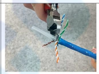
5. Place the conductor pairs into a "star" pattern at a near 90-degree angle to the cable jacket. Cut the cross divider.
